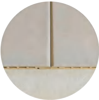
V- seam Splicing
